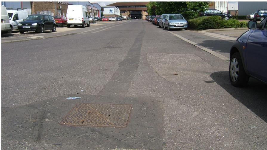
A typical re-instated duct and turning chamber, recently completed by LinchPin.
